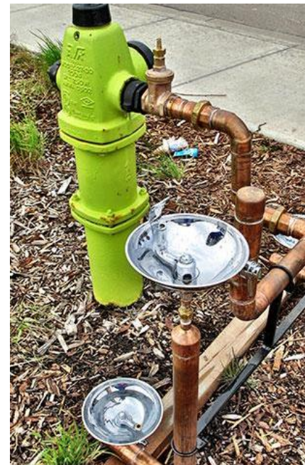
Figure 64. Fire Hydrant Water Fountain by Sans façon. Photo: City of Calgary.
