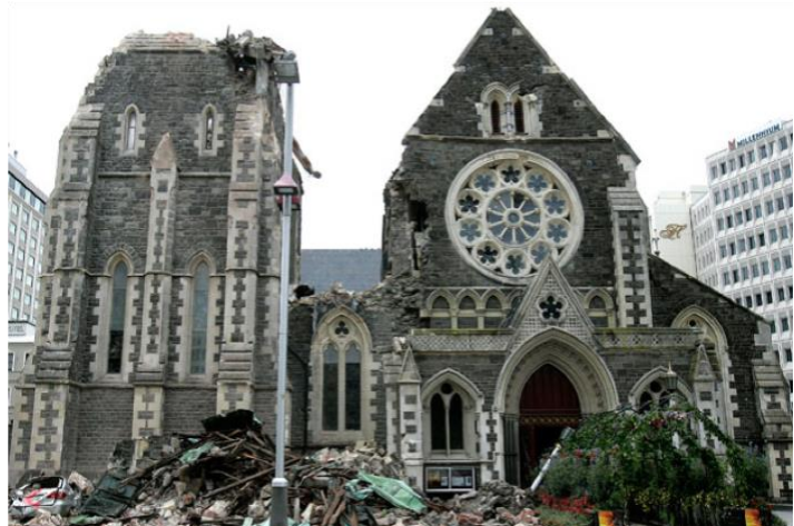
Figure 36. Christchurch Cathedral after the earthquake. Photo: Deborah McCormick.
